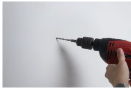
Step 2 Drill the holes at the exit of the wall first.
